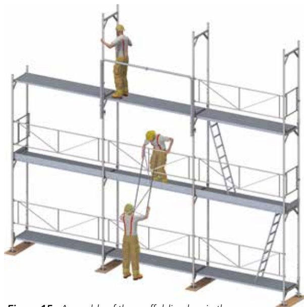
Figure 15: Assembly of the scaffolding bay in the access bay with the protection of the MSG.
