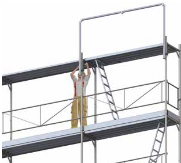
Figure 14: Assembly with the protection of the MSG on the access bay.
