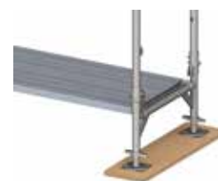
Figure 17: Installation of a safety pin.
